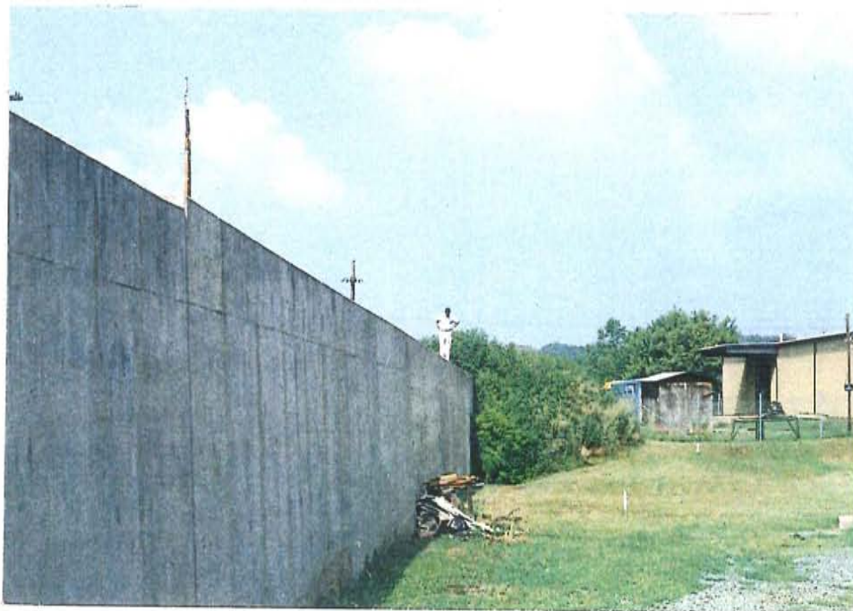
Photo 4-1. Typical section of floodwall
