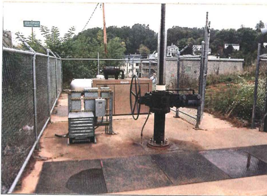
Photo 6-9. On top of levee discharge structure: Emergency generator (background), phase converter (left foreground), sluice gate hand crank (right foreground)
