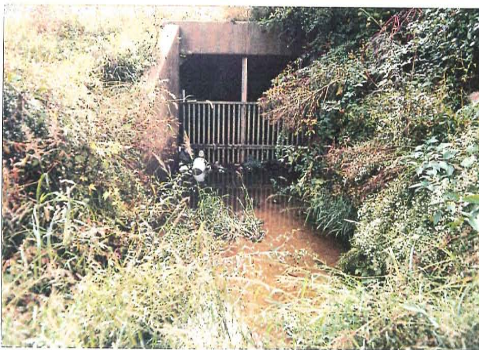
Photo 6-8. Trash rack to levee discharge structure
