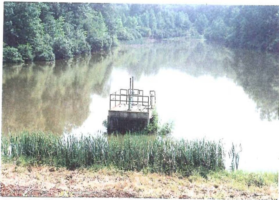
Photo 6-2. Water outlet structure at Mink Creek Dam
